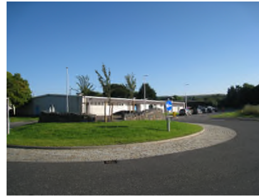
View towards Business Park from Railway Terminus
